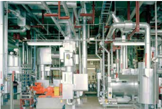
View into Clariant's Licocene plant Einsicht in die Clariant Licocene Produktinsanlage
